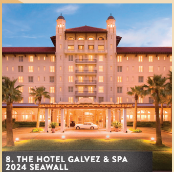
8. THE HOTEL GALVEZ & SPA 2024 SEAWALL
